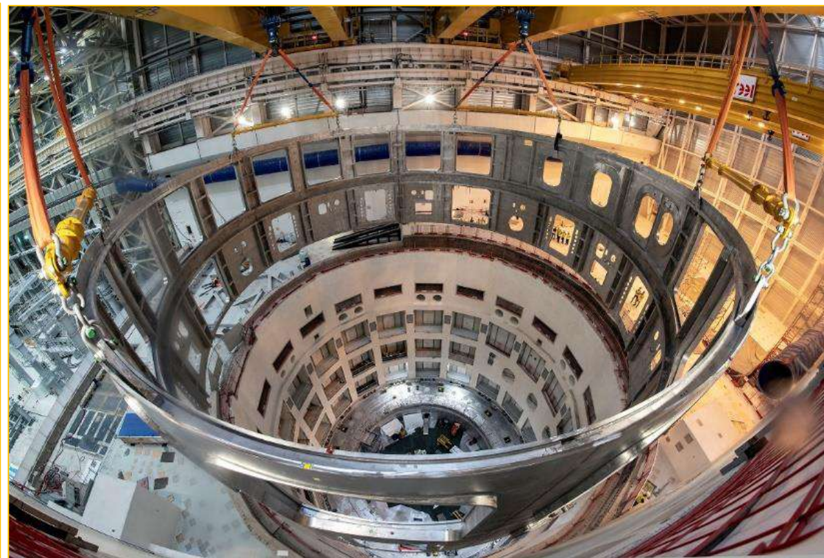
Inserting the Cryostat Lower Cylinder into the Tokamak Pit. Perfect fit with the Base
